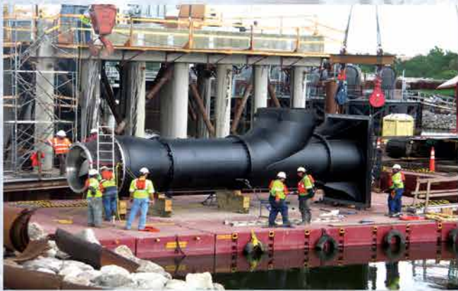
Available in open or enclosed line shaft configurations. Enclosing tubes, when used, are schedule 80 and are supported by spiders when required by the pump length.
