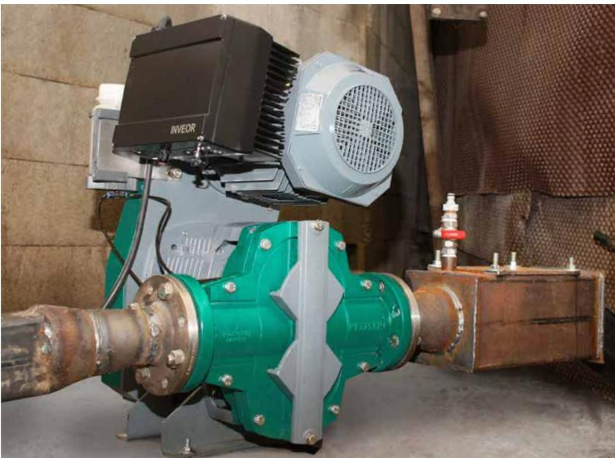
Recirculating liquid manure in a biogas plant from a fermenter to a heat exchanger at a flow rate of 20 m<sup>3</sup>/h against a discharge pressure of 1,5 bar.
