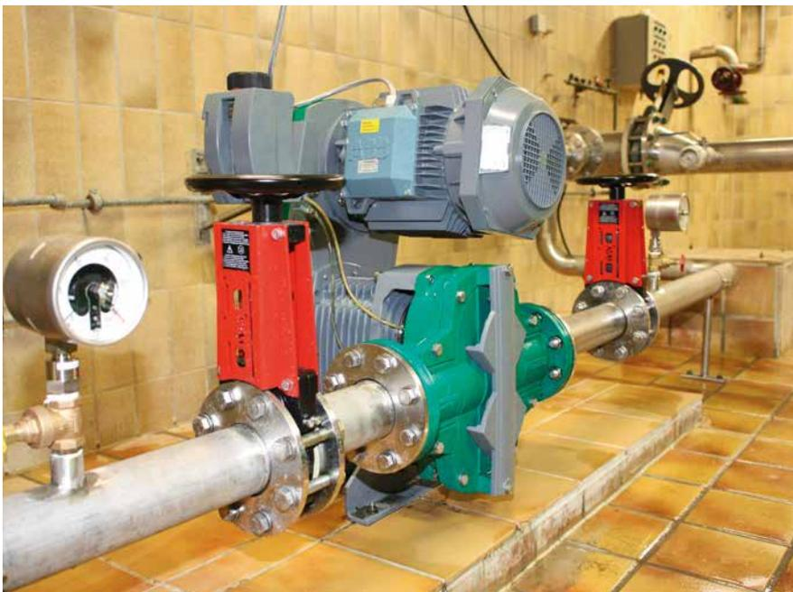
Centrifuge feed: 2 % DS excess sludge at a flowrate of 18 m<sup>3</sup>/h against a discharge pressure of 1,5 bar.
