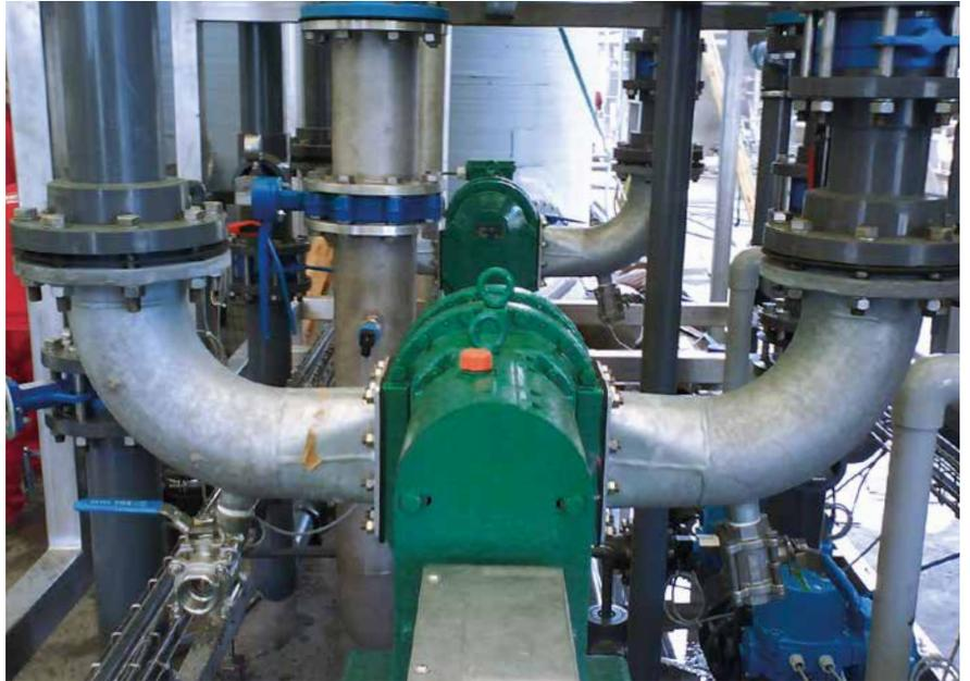
Pumping of water with high content of magnesium ammonium phosphate (MAP): T.Envi® with an annual conveying volume of approximately 22,000 m<sup>3</sup>/h.
