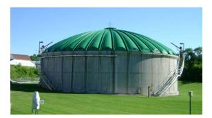
A fiberglass dome cover at a local wastewater treatment plant was in desperate need of repair. It showed signs of delamination and deterioration - common problems when exposed to the elements.
