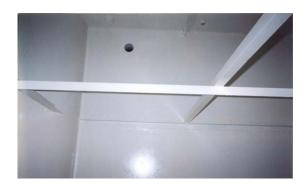
After years of service, the corrosive effects of this food ingredient had taken its toll. The tank needed a new lining. During a scheduled down, and under confined space requirements, Crane Engineering got to work.
